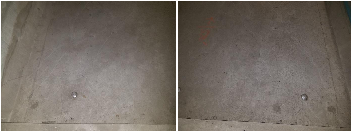
Figure 4 Diagonal cracks across box floor originating from floor/web interface just beyond post tensioning anchorage
