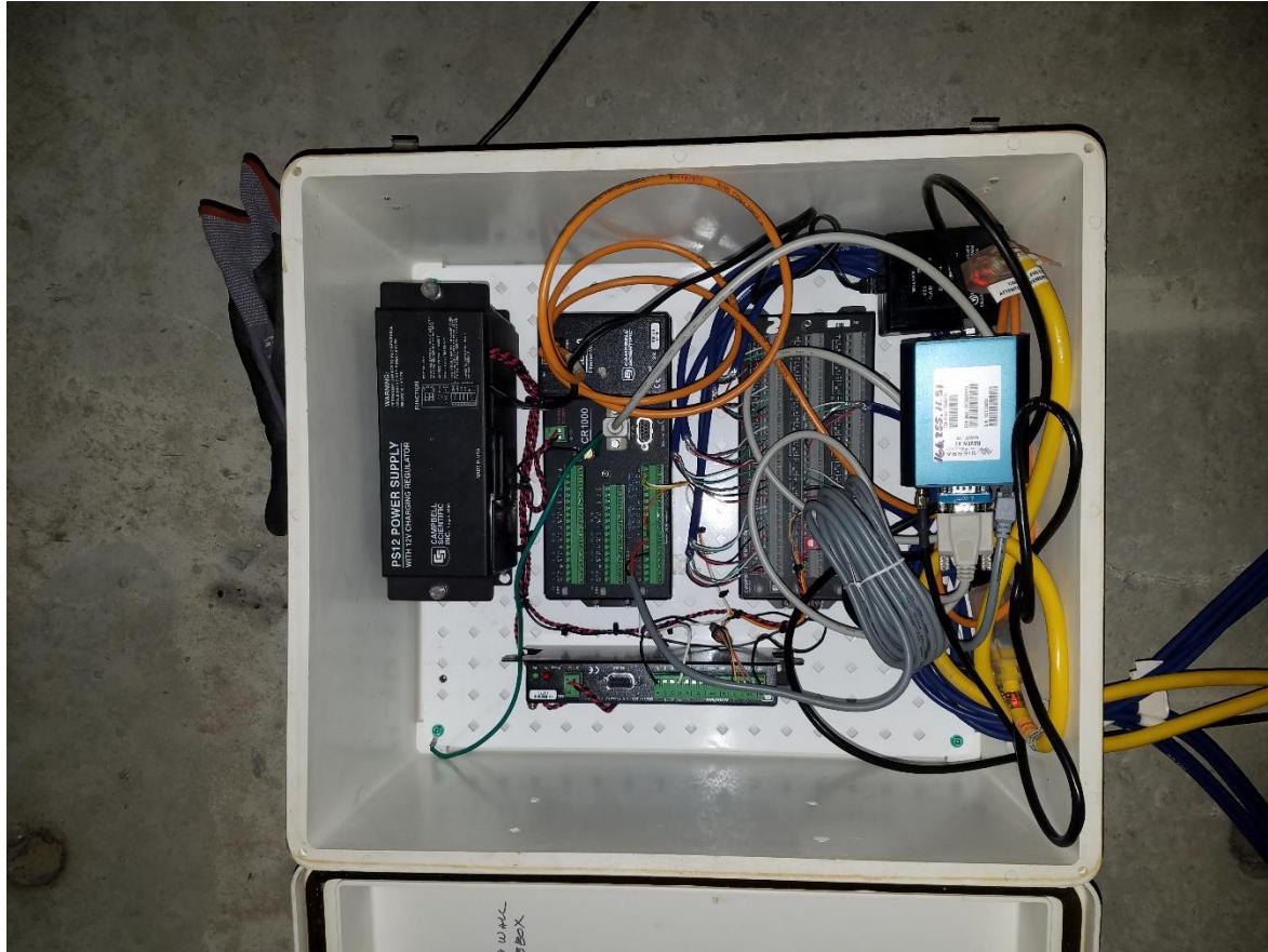
Figure 2 Existing logger cabinet consisting of CR1000 logger, AM16/32 multiplexer, RavenXT modem, AVW200 VW
