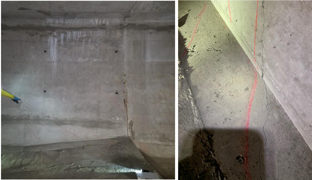
Figure 5 Diagonal shear cracks on box webs and at floor/web interface
