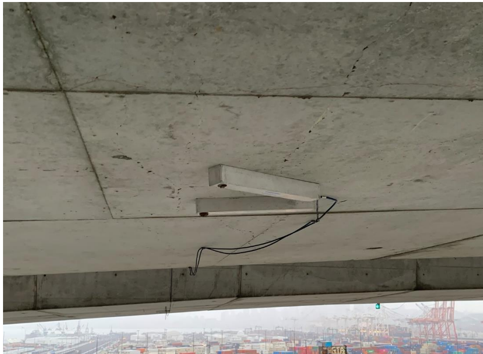
Figure 3 Typical crack meter installation on soffit of box girders
