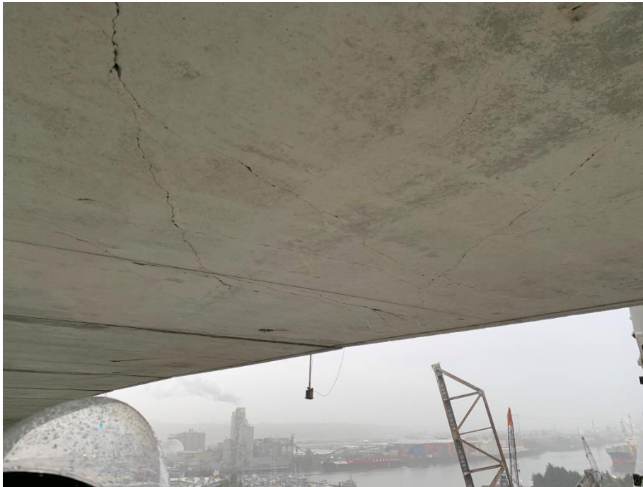
Figure 8 Bottom flange diagonal cracks shifting to transverse cracks near middle of box girder.
