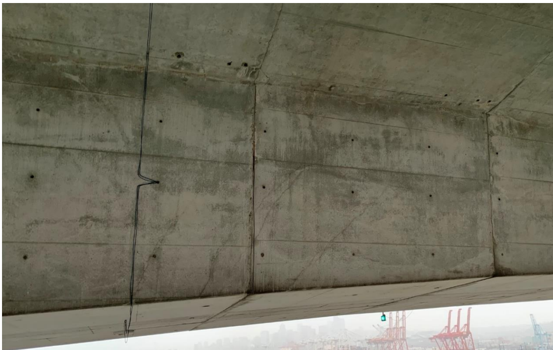
Figure 7 Diagonal shear cracks in exterior face of vertical web.
