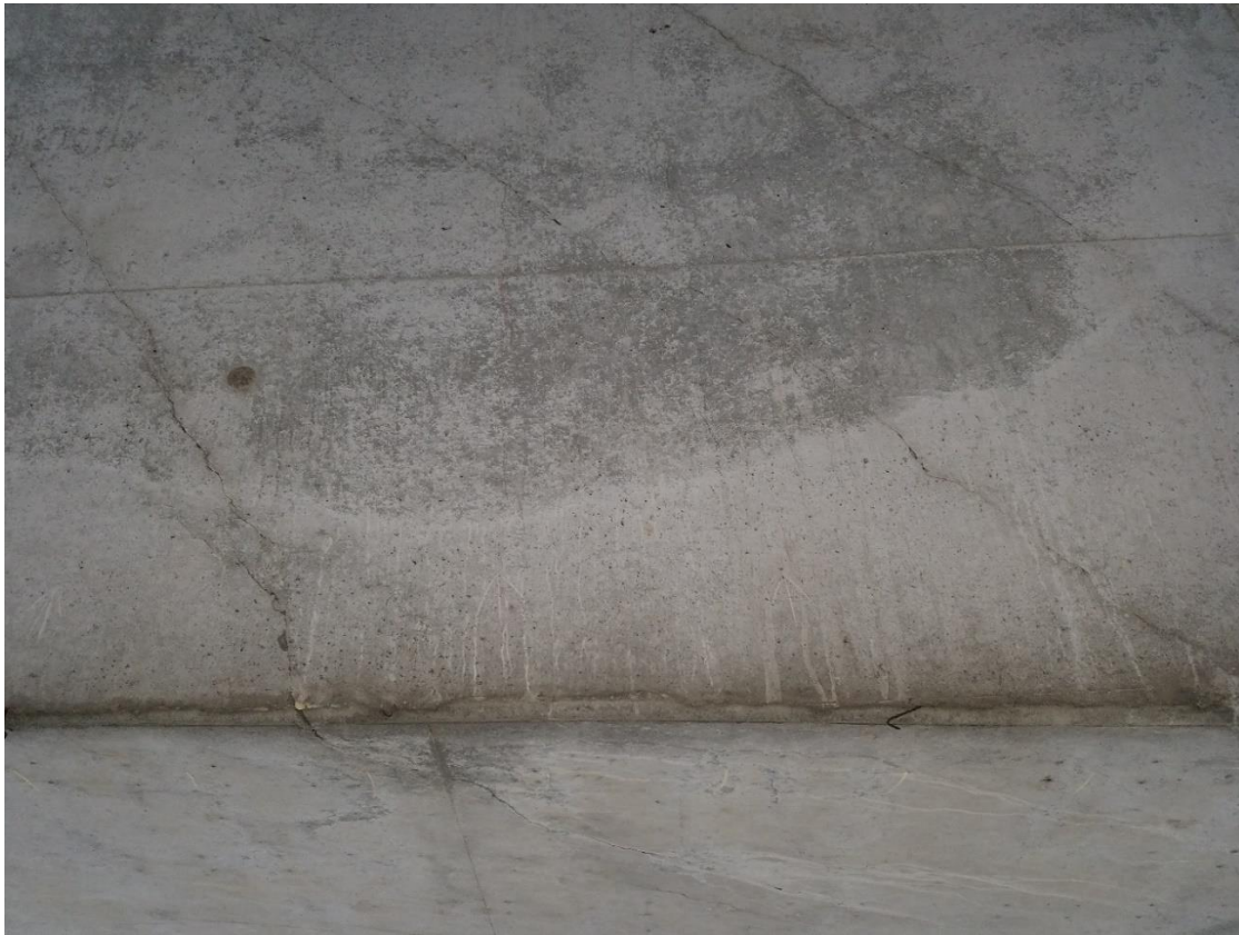
Figure 6 Continuation of bottom flange diagonal cracks into web – exterior bottom flange / web interface.
